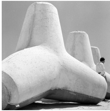
Standard conventional concrete tetrapod (right) and EConcrete tetrapod (left) Source: EConcrete
